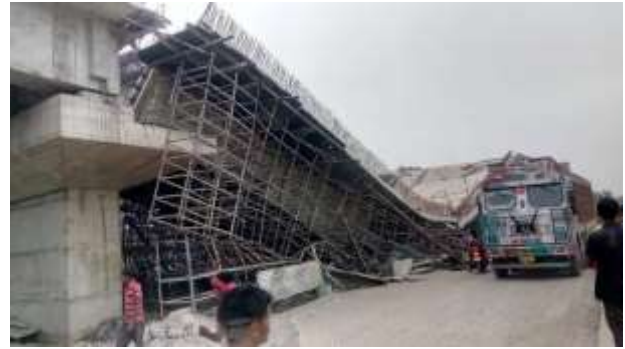
Figure 2 Slab of Under-construction Flyover
