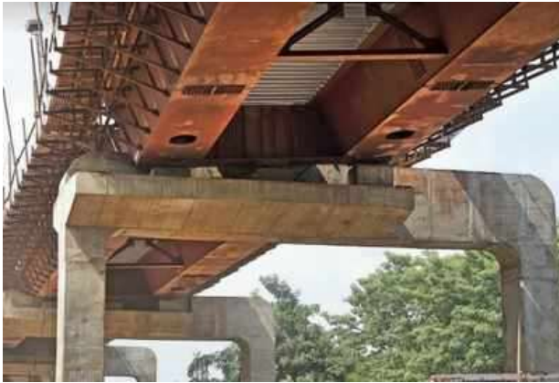
Figure 5 Foundation of Flyover
