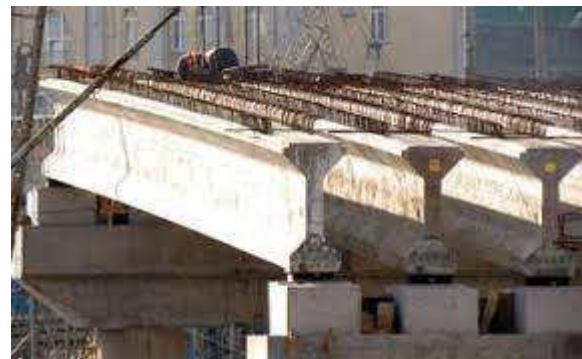
Figure 3 Beams of Flyover
