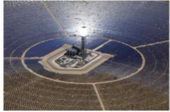
Figure 5 130 MWel Central receiver power plant close to Las Vegas in the US. Brightsource Energy
