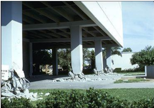
Fig. 1: Examples of failure of buildings with soft storey at ground floor
