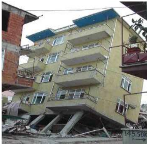
Fig. 1.1: examples of failure of buildings with soft storey at ground floor
